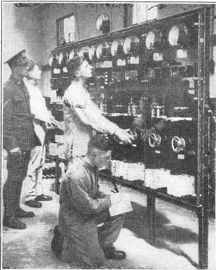
The control panel of the generating plant in the power house.
